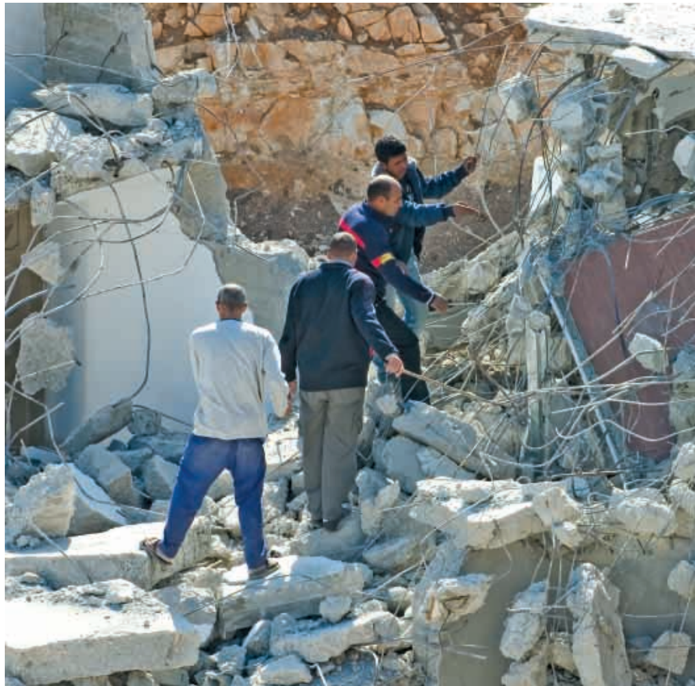
Minutes after a house demolition on the Mount of Olives December 2006, by B. Madsen
