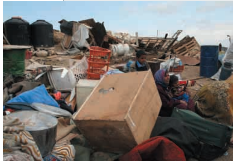
House demolition in Jahalin Bedouin Camp February 2007 K.Johansson
