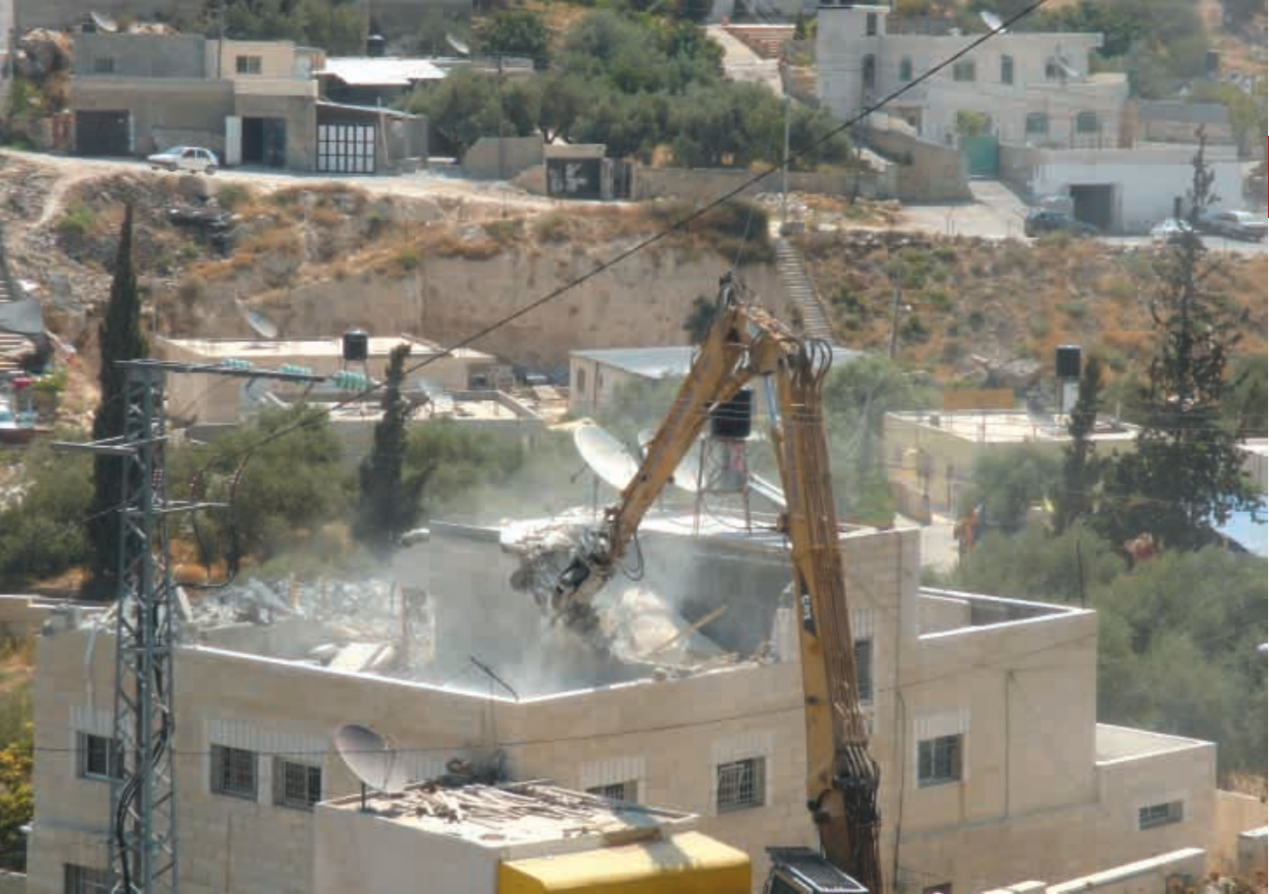
House demolition in Jerusalem July 2007, by P. Mukerji
