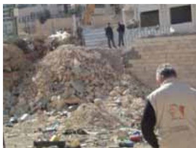
Ecumenical Accompanier, Osten Gunnarsson inspecting the wreckage of a demolished house in East Jerusalem.
