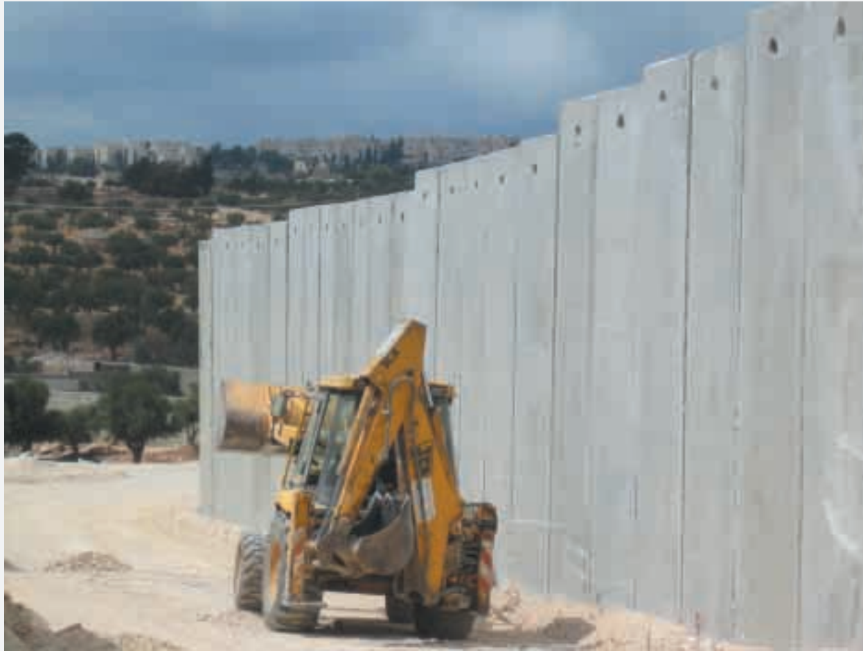
Construction of the Wall Continues
